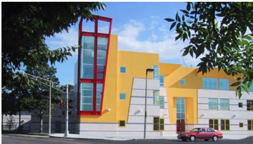
Stull and Lee, Orchard Gardens School, photo courtesy of architect
